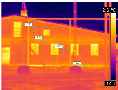
Figure 6. East façade of piggyery (part 1)
